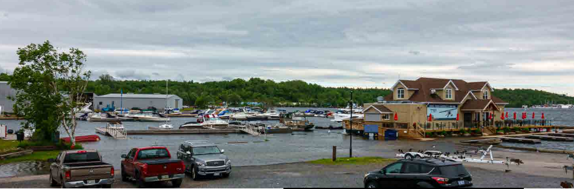
High water in the Parry Sound harbour in June 2020.
