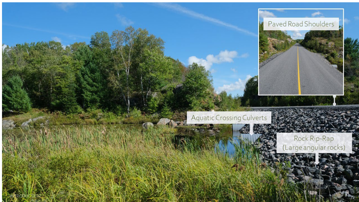
Figure 3. Example of alternative mitigation strategy for reducing road threats to local turtle communities (Figure from Kentel, 2023).
