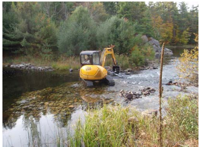
Figure 6 – Excavator placing and manipulating rock present at and imported to the site
