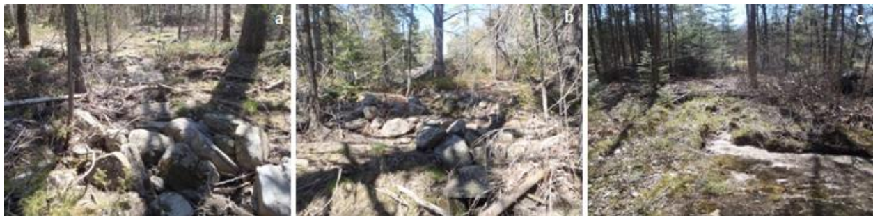
Figure 8. Young's Rapids bypass channel: (a) and (b) rocky portion of the channel; (c) bottom of bypass channel where sediment and grass have covered the former bedrock base of the channel.
