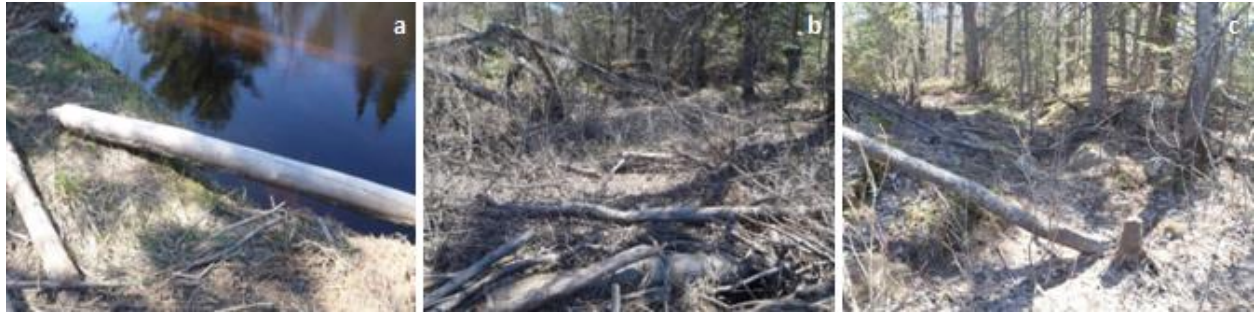
Figure 7. Young's Rapids bypass channel: (a) top of the channel that has filled in over many years; (b) looking down the bypass channel from the top at the material that has filled in over time; (c) immediately below the blocked area where the channel is still somewhat defined.
